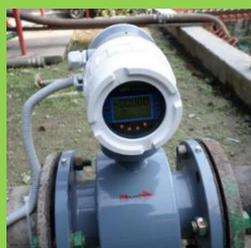
**Electronic smart meters** are the preferred option because they can relay their information to central monitoring and control units. These electronic meters are more expensive than turbine or mechanical meters but they are more accurate and have the advantage of removing 'human error' because the 'steps' of hand written log books and transcription of data into spread sheets are omitted.
